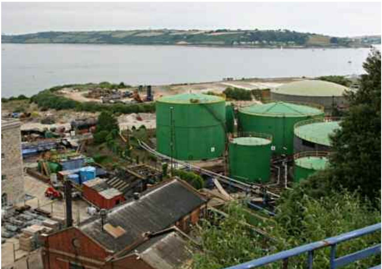
Figure 8 Oil storage tanks at Falmouth docks, Cornwall, in south-west England. Note the occupied buildings adjacent to the storage tanks, and the estuary which leads into the English Channel
